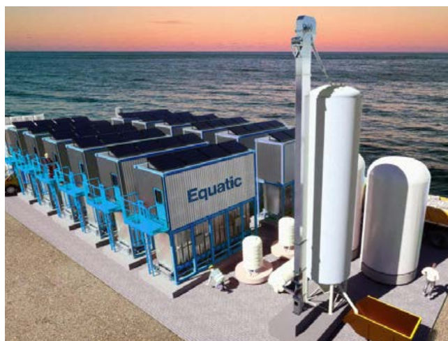
An illustration of Equatic's next project: a larger, pre-commercial carbon direct removal and hydrogen generation plant. EQUATIC
